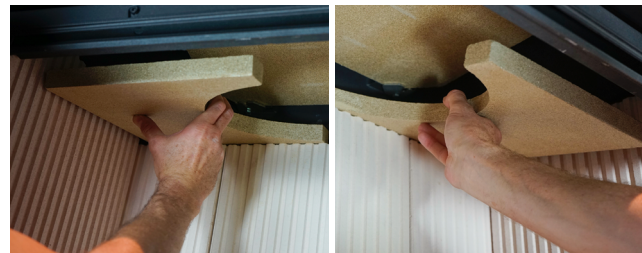
Removal of lower deflector plates. (HKD13)
