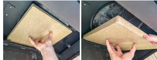
Removal of upper deflector plate
